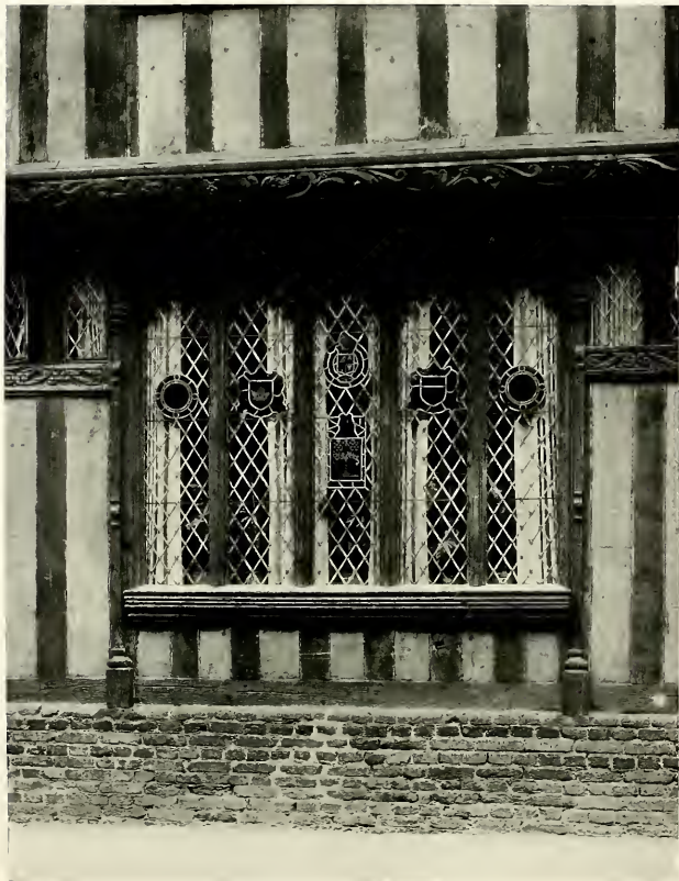
OLD OAK HOUSE, DETAIL OF WINDOW Only the small windows at either side open
